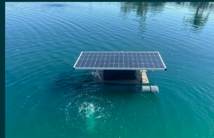
Floating-photovoltaic (FPV) power on a floating island, with battery back-up; powering a submerged NB generator.
